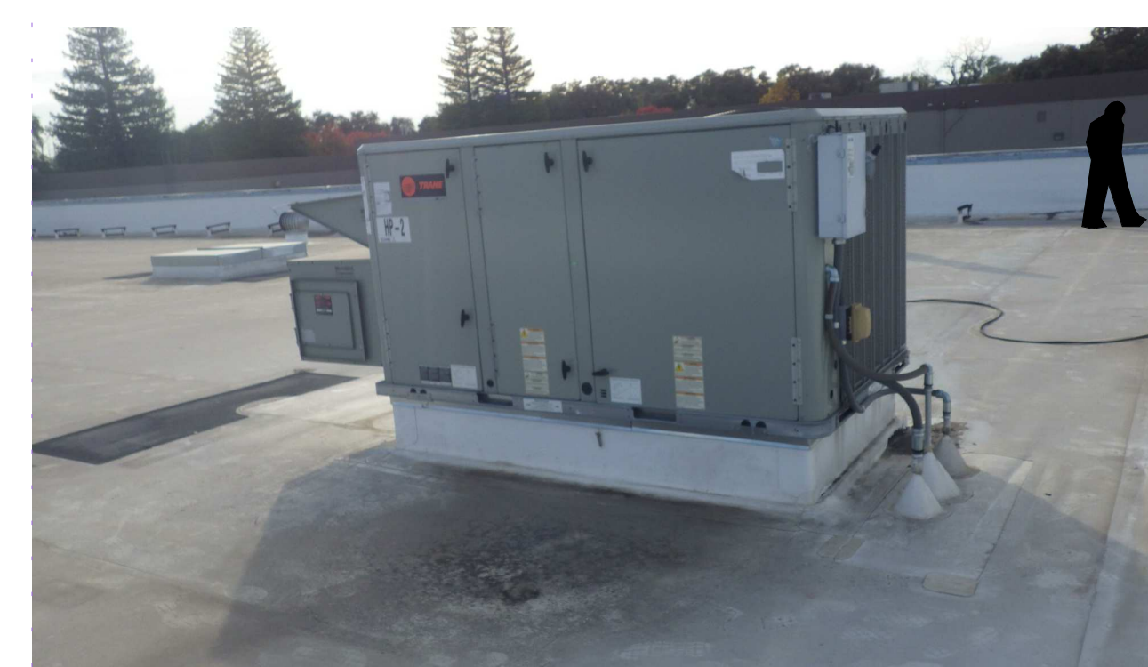
UNIT A EXISTING HVAC UNIT, PIPE, & CONDUIT PENETRATIONS TO REMAIN
