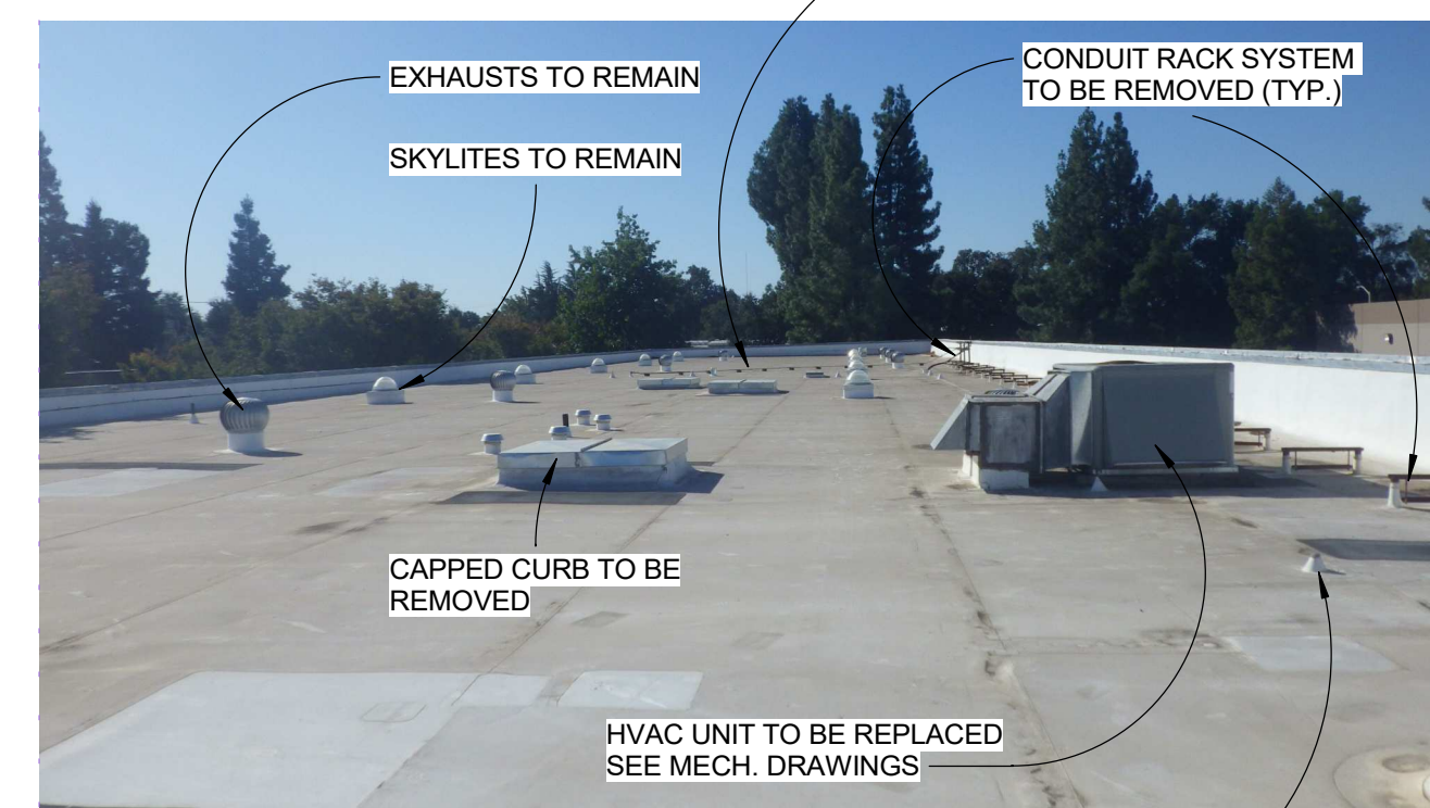
9 (E) ROOF OVERVIEW FROM NORTH END 12" = 1'-0"
