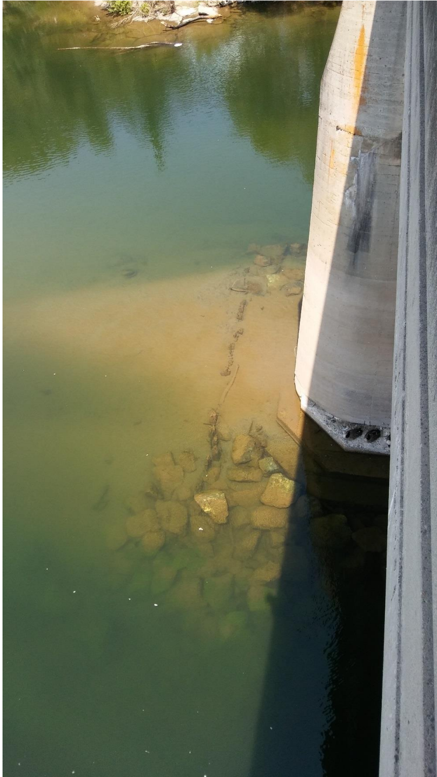
Figure 4. 4 – Example of the existing rock slope protection that will be removed and replaced with new permanent sheet piles. Some of the existing rock slope protection has been carried away while some remains in place. This photo is showing the downstream portion of the pier.
