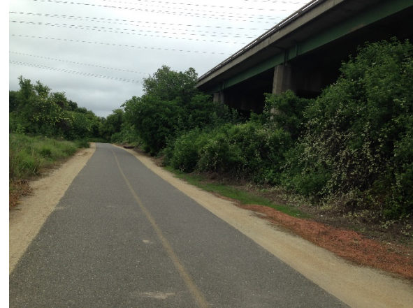
6: GROUND LEVEL PHOTO LOOKING AT EXISTING BIKE PATH UNDER SR 51.
