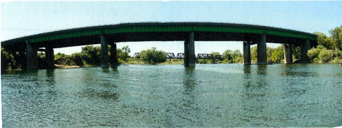
Photo 2 – American River Bridge, Br. No. 24-0003
