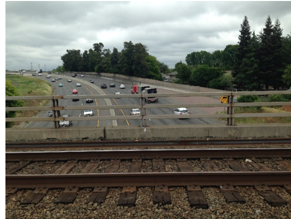
2: GROUND LEVEL PHOTO LOOKING TOWARDS SR 51 FROM UNION PACIFIC RAILROAD UNDERCROSSING.
