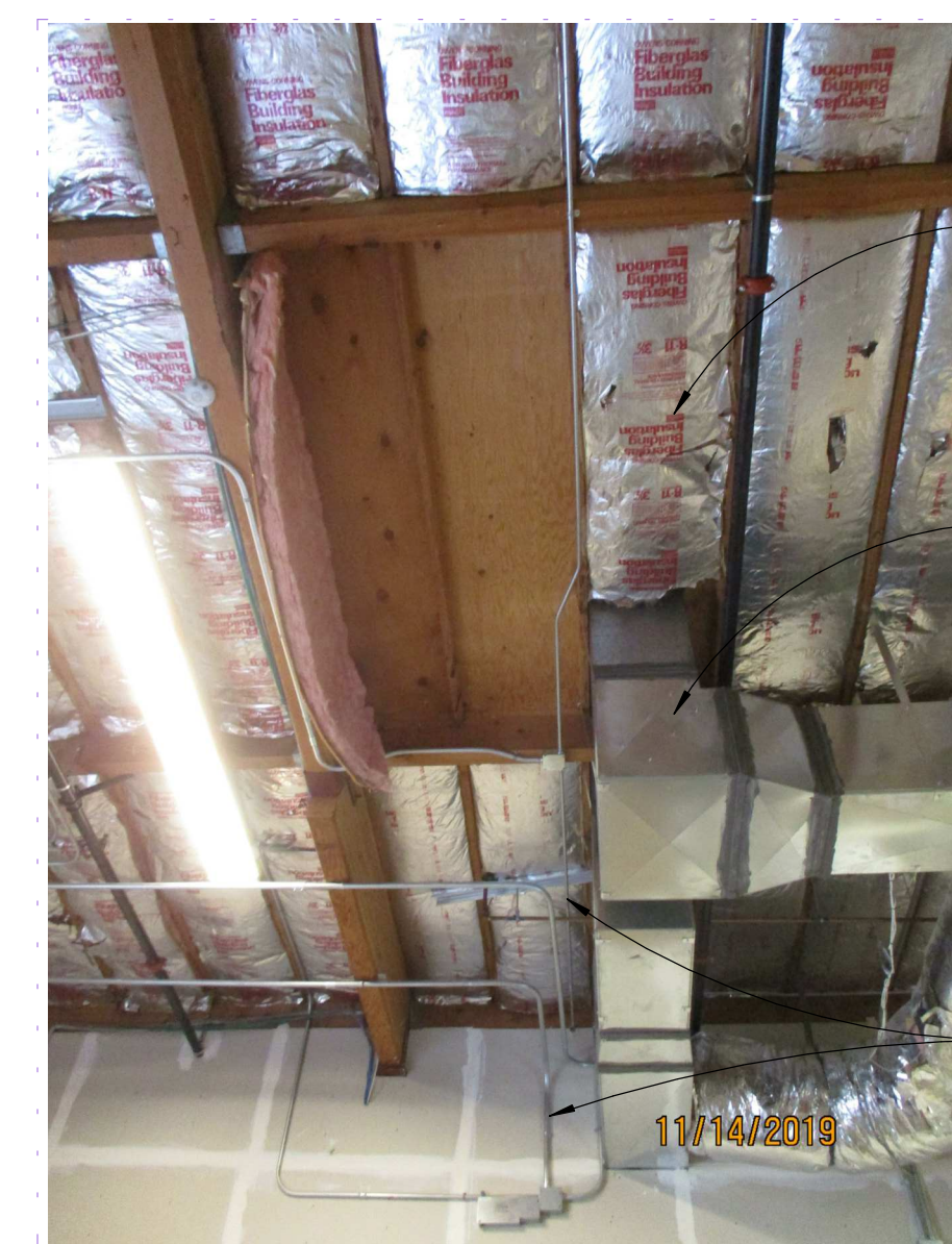
5 CEILING AT MECH UNIT B
