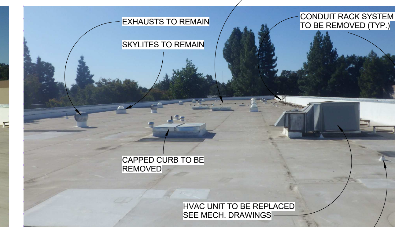
9 (E) ROOF OVERVIEW FROM NORTH END 12" = 1'-0"
