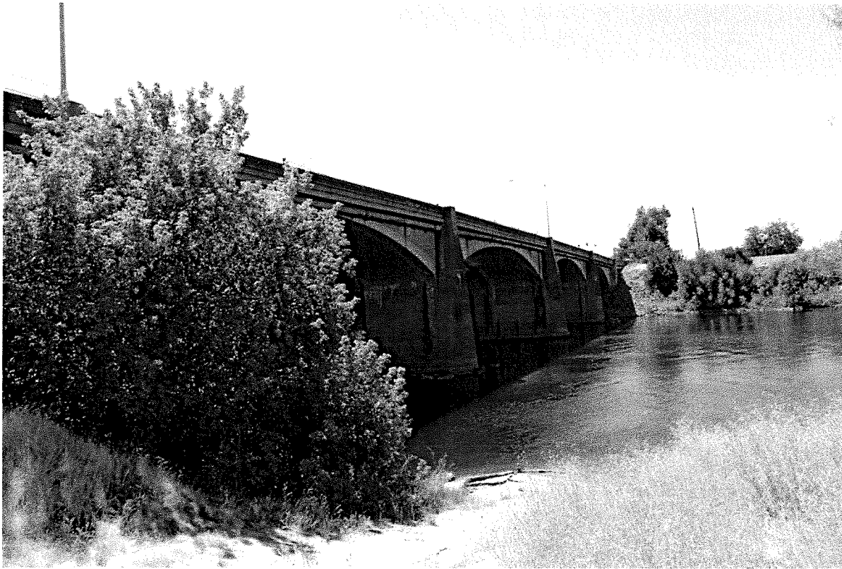
Figure 4. 3 - View of the 12 th Street Bridge on state route 160 across the American River from the west side. This view is looking south. The south bank, where the federal levee is located, has existing rock slope protection. Also seen is the existing north bank which does not feature a levee.
