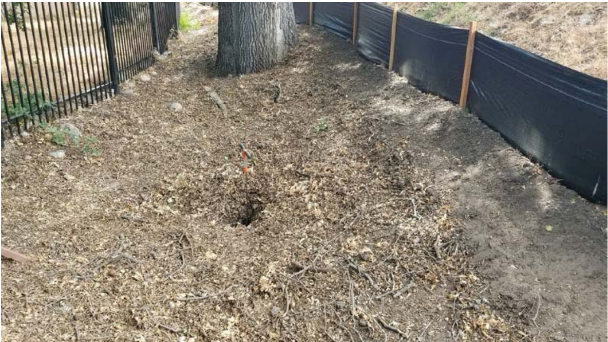
Figure 3. 18" CMP culvert along landside slope looking west
