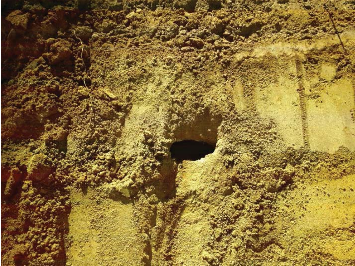
Figure 4. Closeup of 18" CMP culvert along waterside slope
