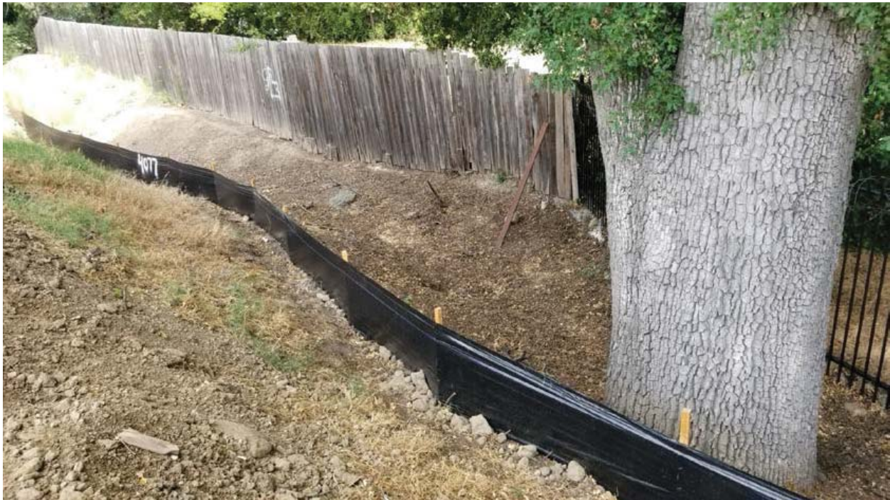
Figure 1. Landside slope on Arcade Creek south levee looking southeast
