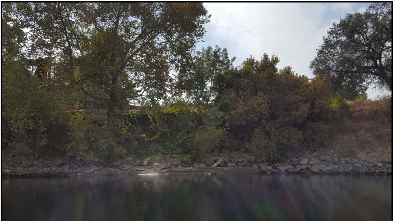
Photograph 22 - LAR RM 2.7L (1), upstream of repair site
