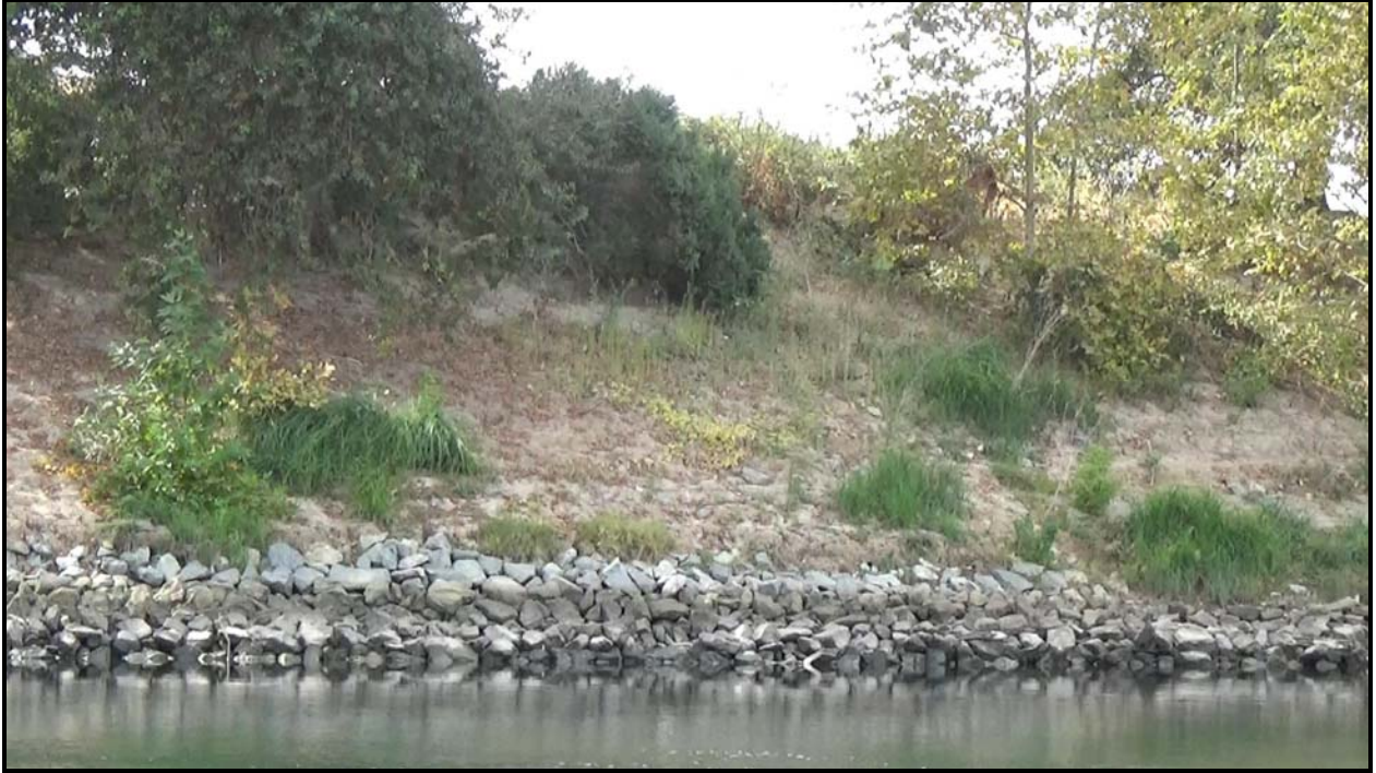
Photograph 23 - LAR RM 2.7L (2), repair site
