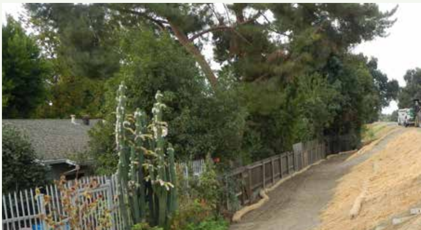
The American River Flood Control District redesigned the levee section, removed the dirt, and built a wide gravel path behind 15 properties, including the Giordano's.
