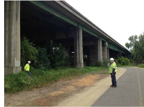
8: GROUND LEVEL PHOTO LOOKING TOWARDS AMERICAN RIVER BRIDGE FROM THE EXISTING BIKE TRAIL
