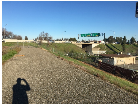
4: GROUND LEVEL PHOTO LOOKING TOWARDS TRIBUTE ROAD OVERCROSSING FROM THE RIVER LEVEE.
