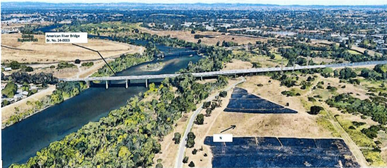
Photo 1 - Aerial view of the American River Bridge, Br. No. 24-0003
