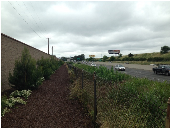
3: GROUND LEVEL PHOTO LOOKING AT MCKINLEY SOUNDWALL AND NB SR 51.
