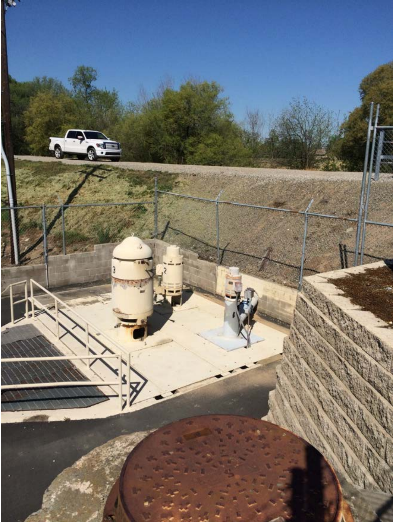
Figure 1: Sump 159 looking North West
