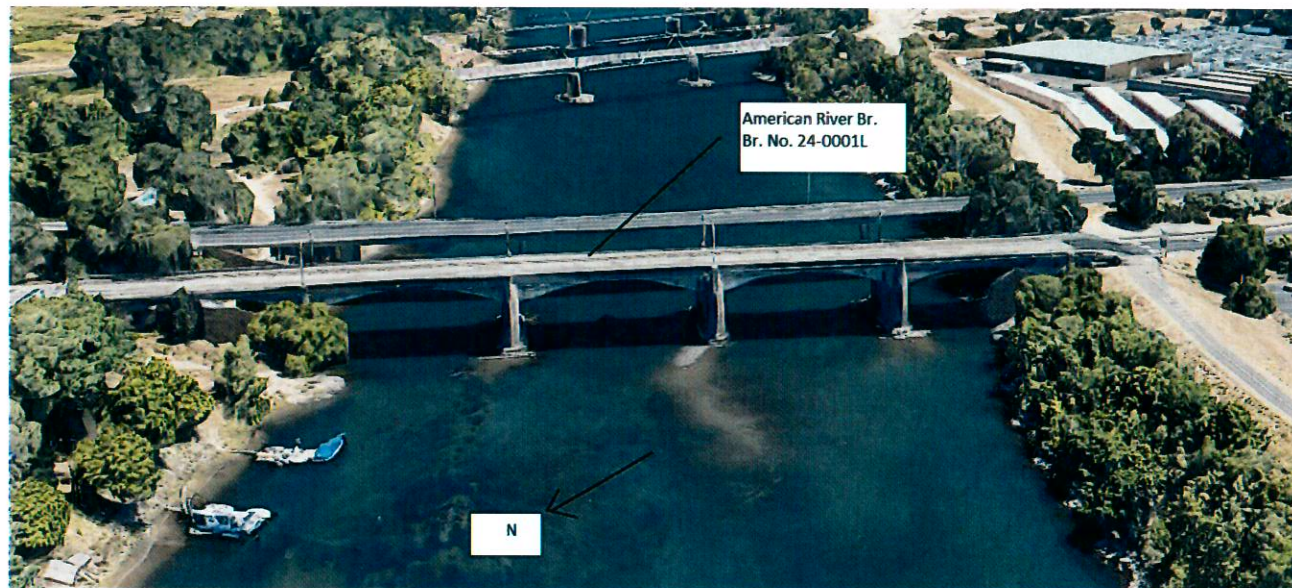
Figure 1- American River Bridge, Br. No. 24-0001L on SR 160
