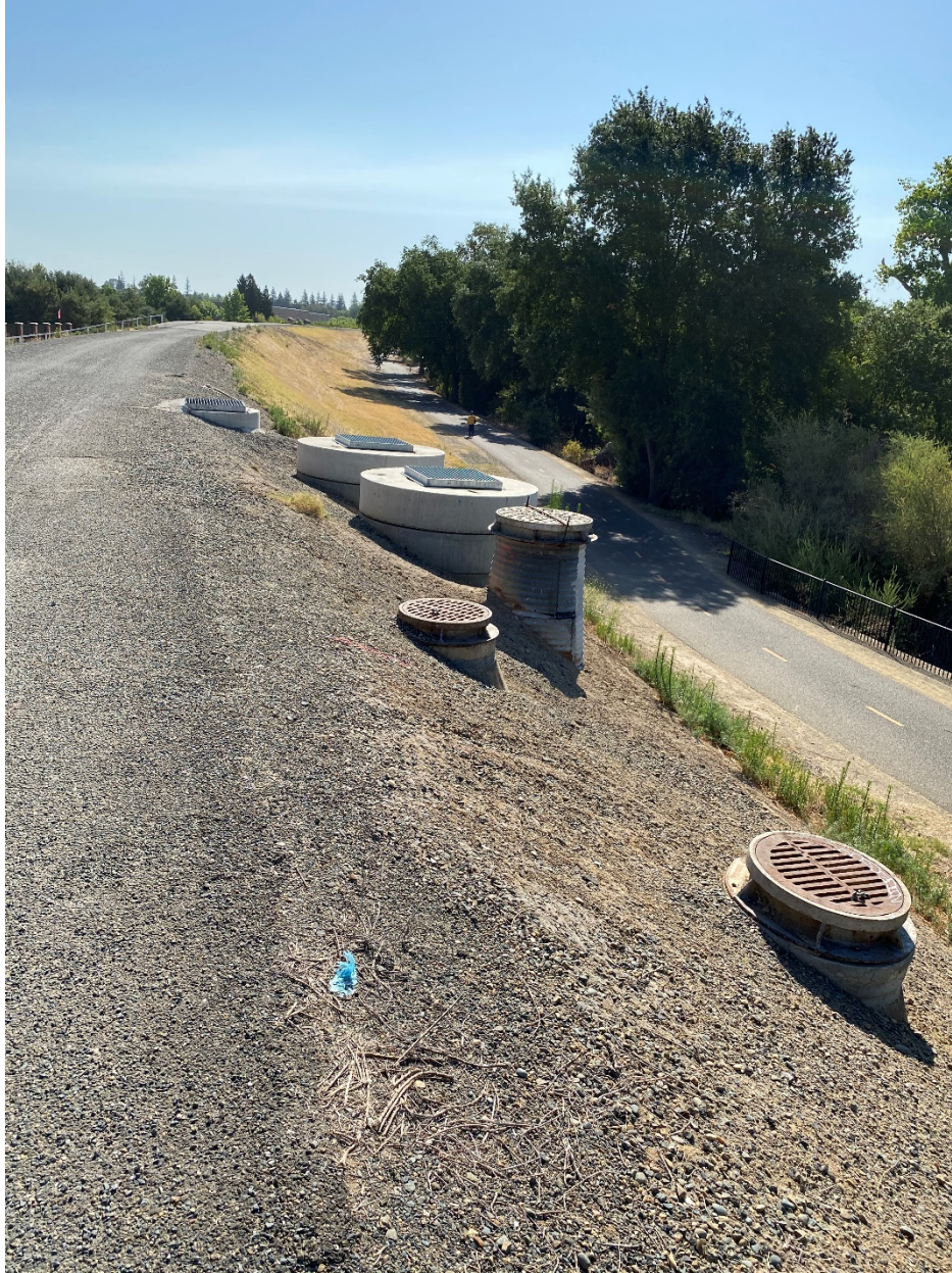
Figure 3: View from crest of Levee facing eastward
