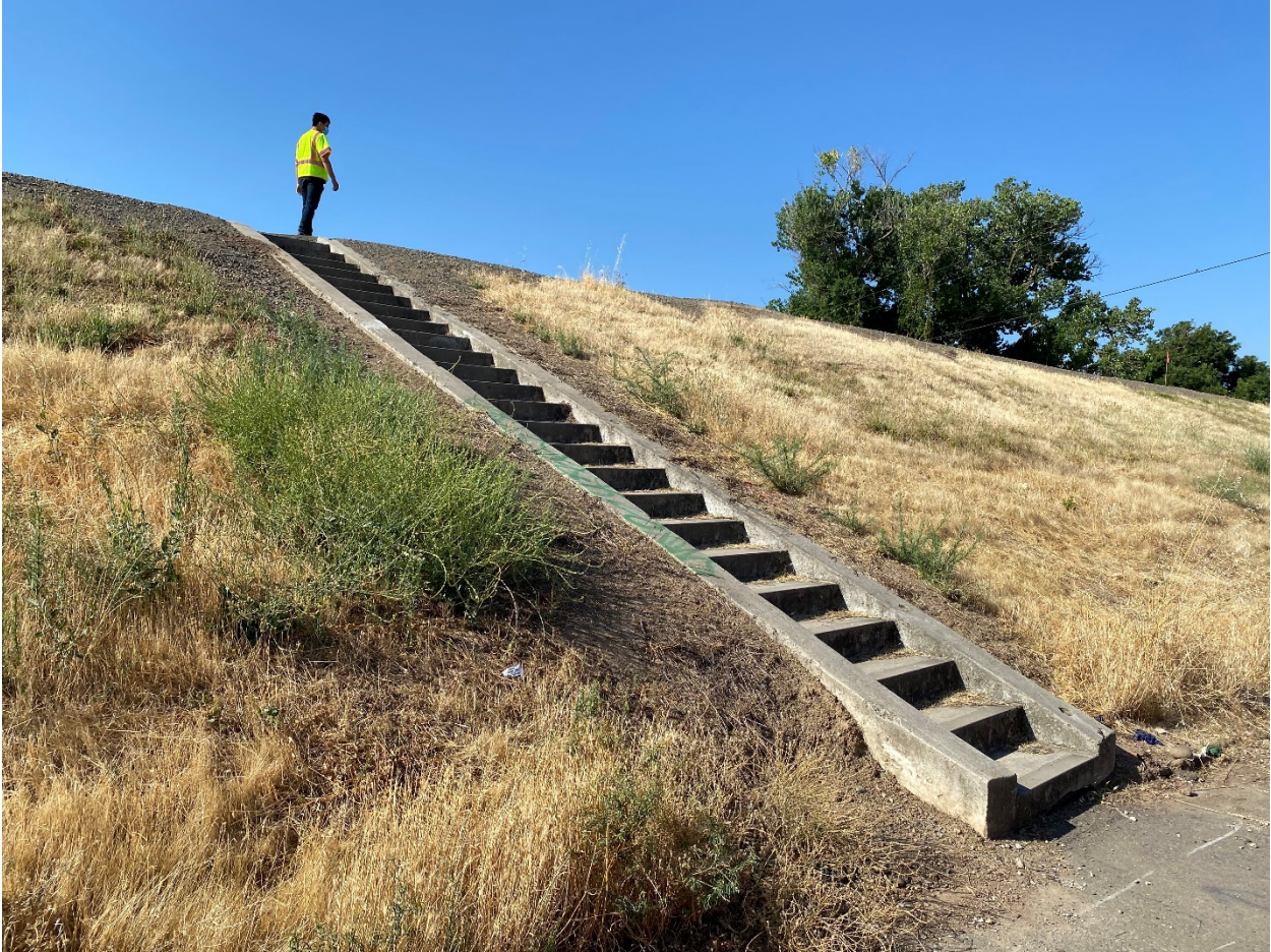
Figure 2: View of landside levee slope
