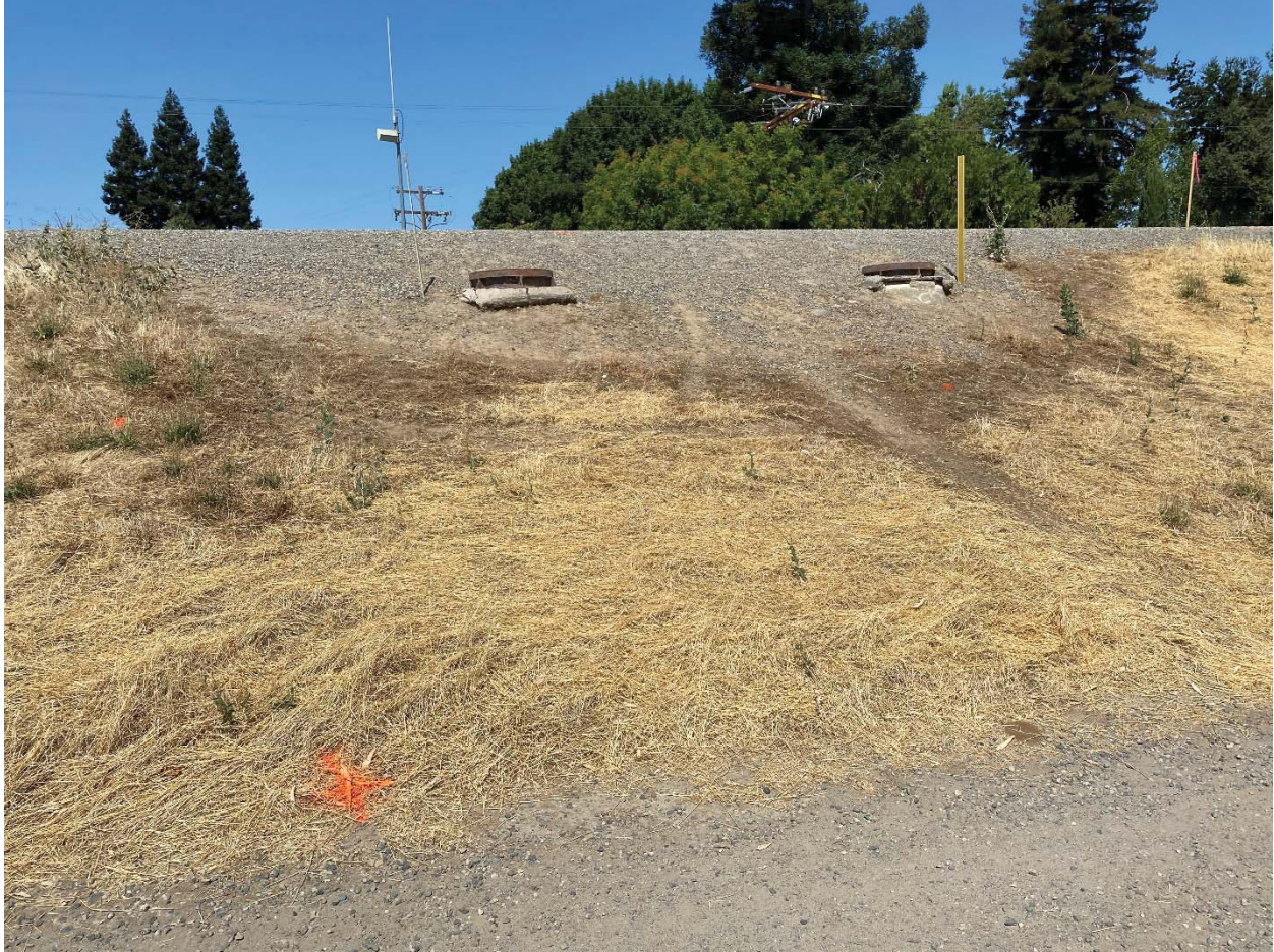
Figure 2: View from waterside TOE of Levee facing Levee crest (upstream)
