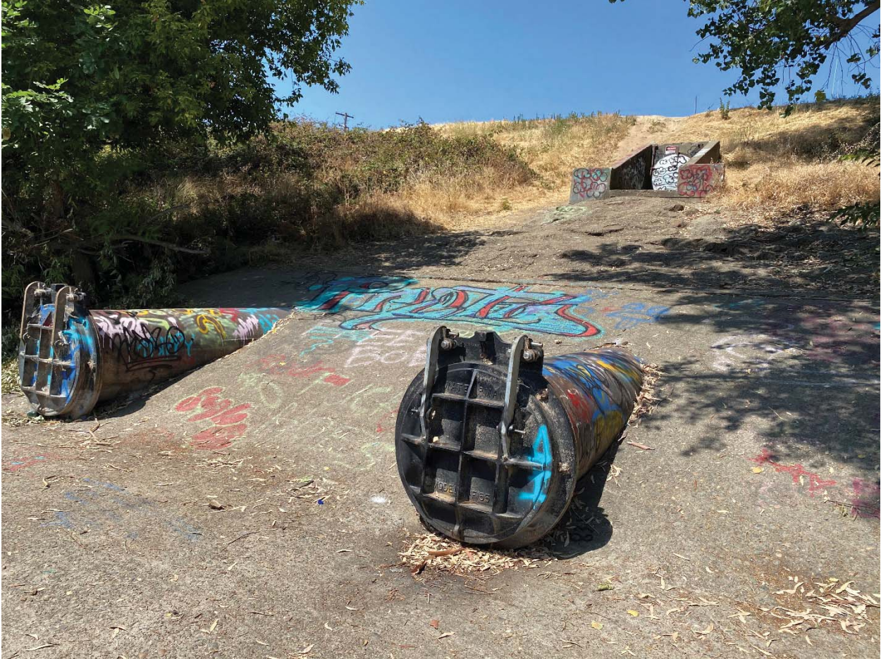
Figure 4: View of outfall structure with flapgates at the waterside slope of Levee
