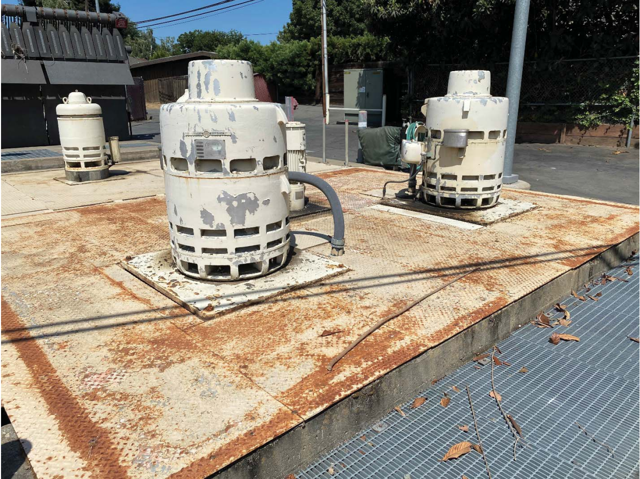
Figure 1: View of pump station
