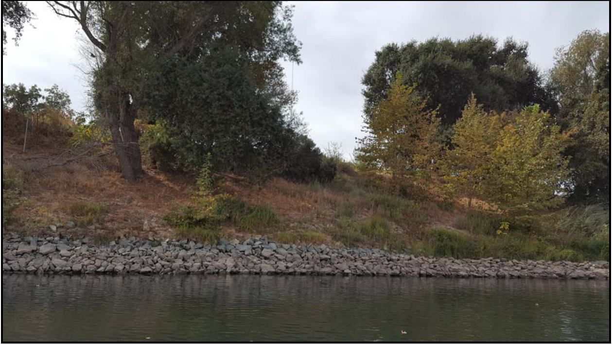
Photograph 21 - LAR RM 2.7L (2), repair site
