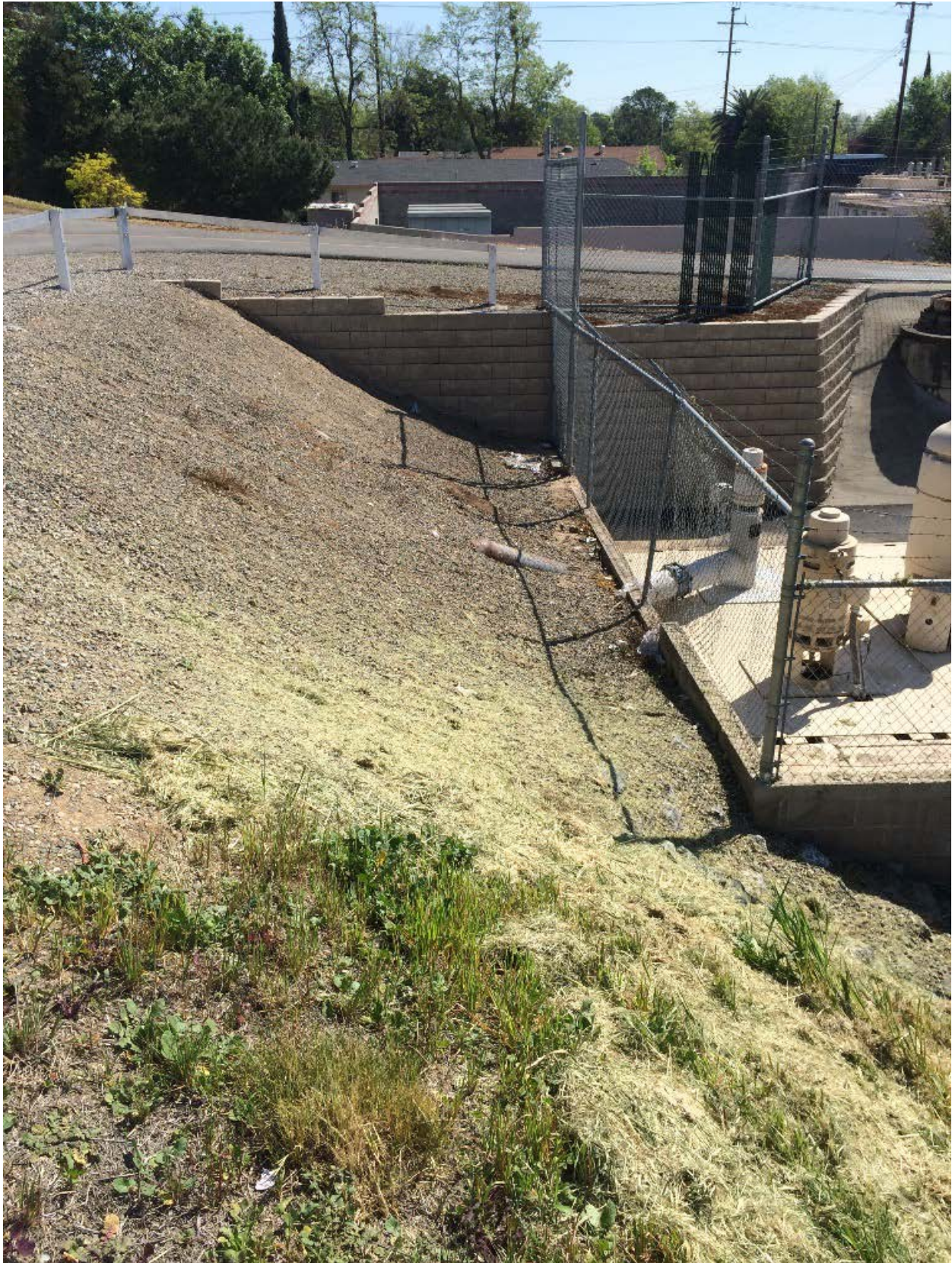
Figure 2: Landside slope near Sump 159
