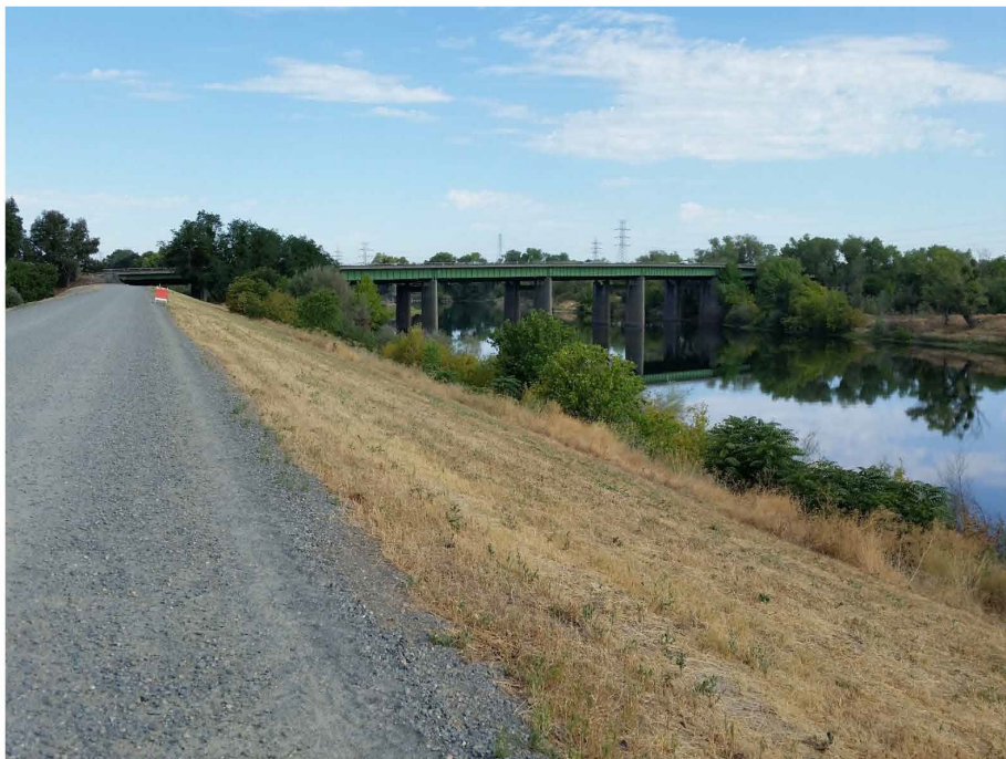
Facing west towards Business 80 bridge. The proposed trail would be on the top of the levee here due to the lack of a levee toe road.
