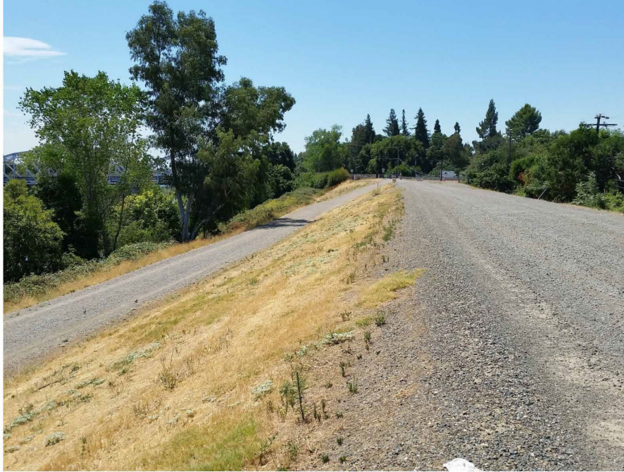
Facing east toward connection to existing trail at H Street.
