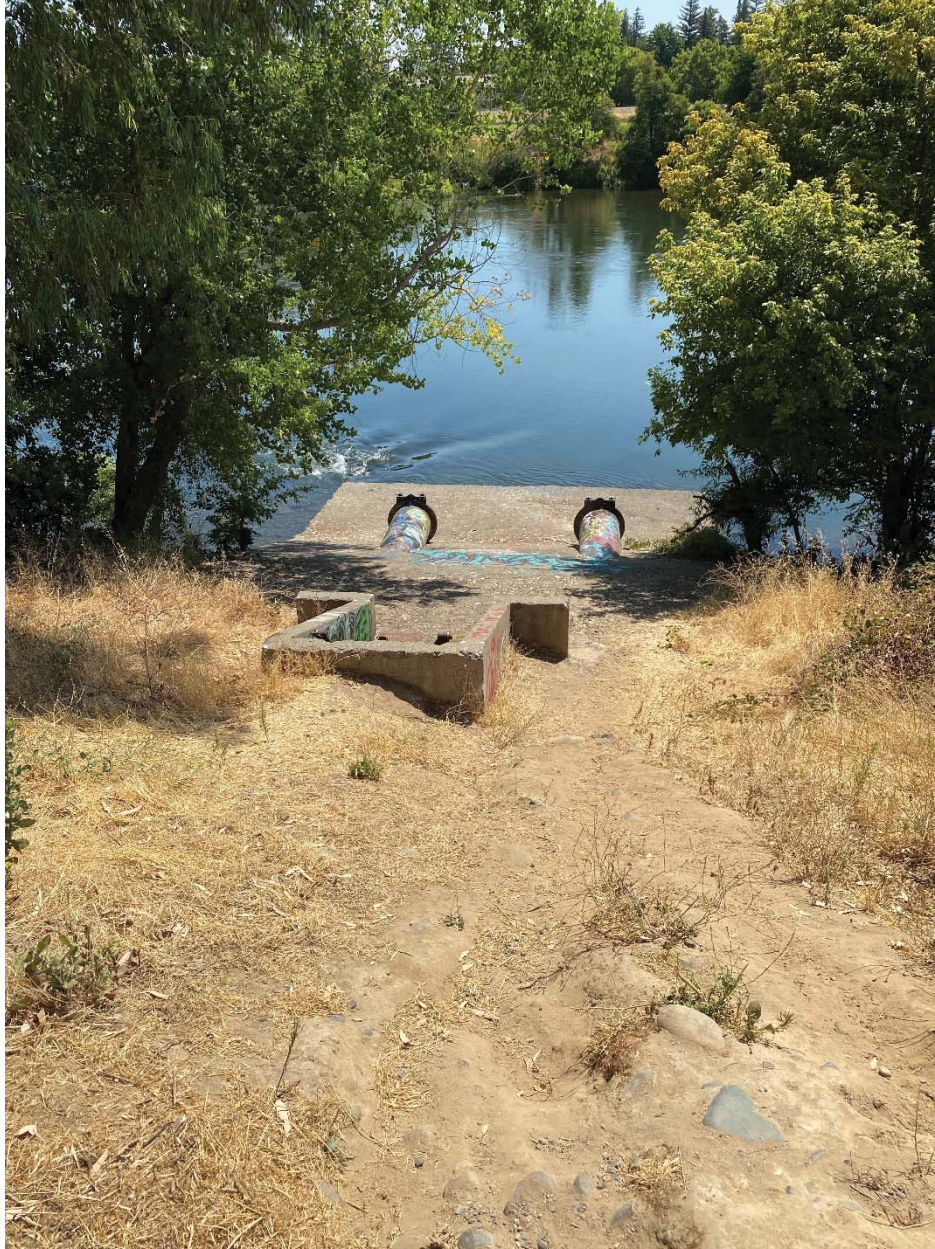
Figure 3: View from waterside slope of levee facing downstream towards American River
