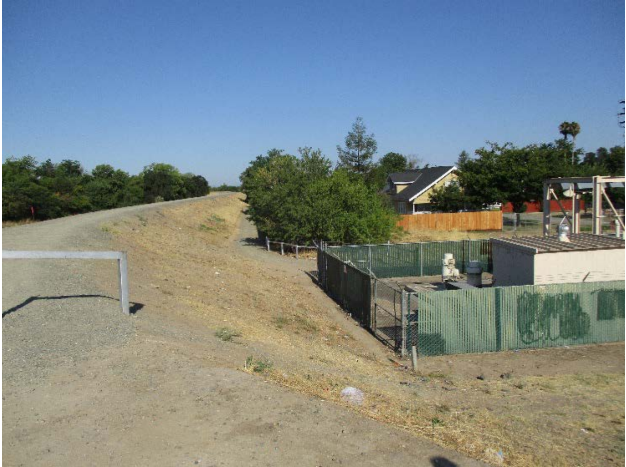
Figure 2: View looking west on the land side of the levee.
