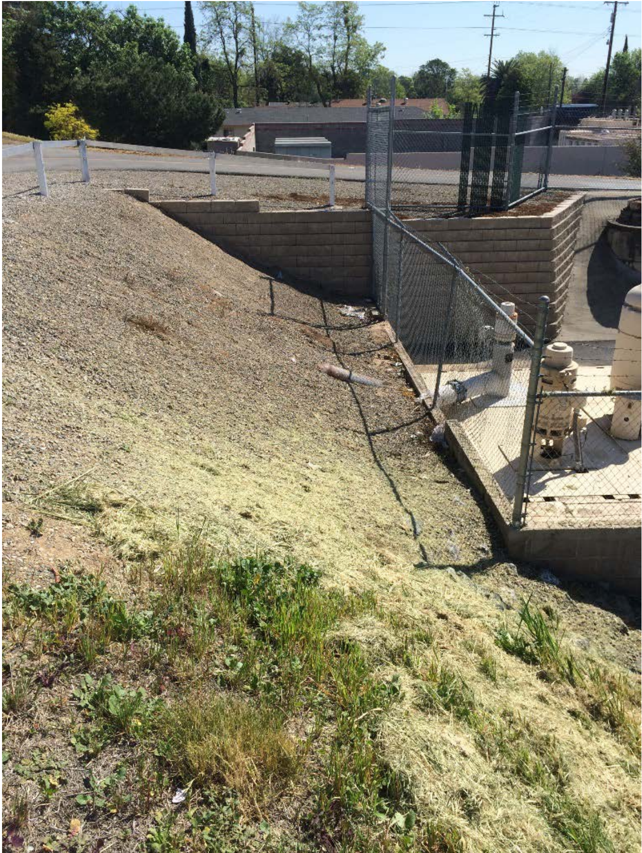
Figure 2: Landside slope near Sump 159
