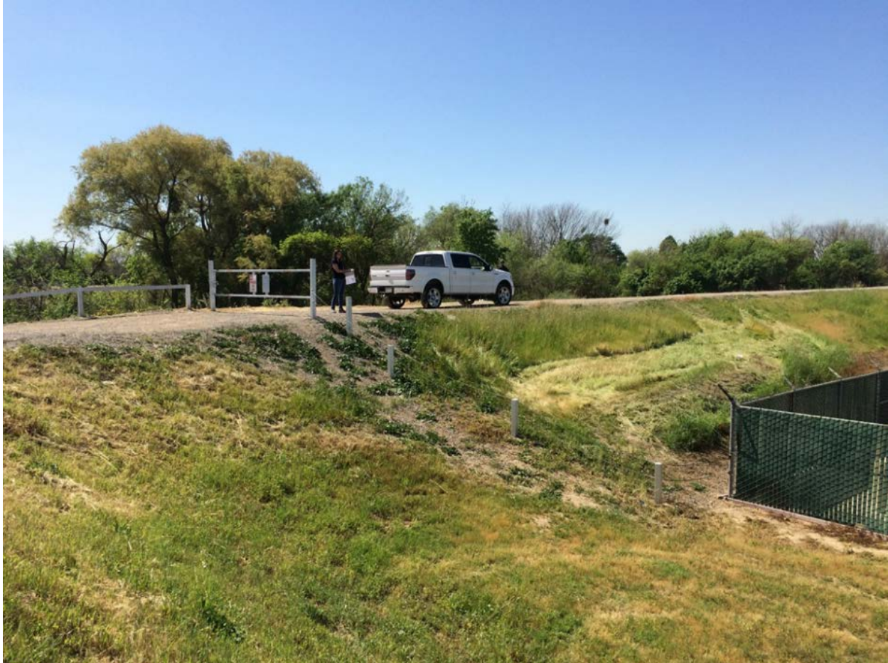
Figure 1: Arcade Creek north levee near Sump 103 looking south west
