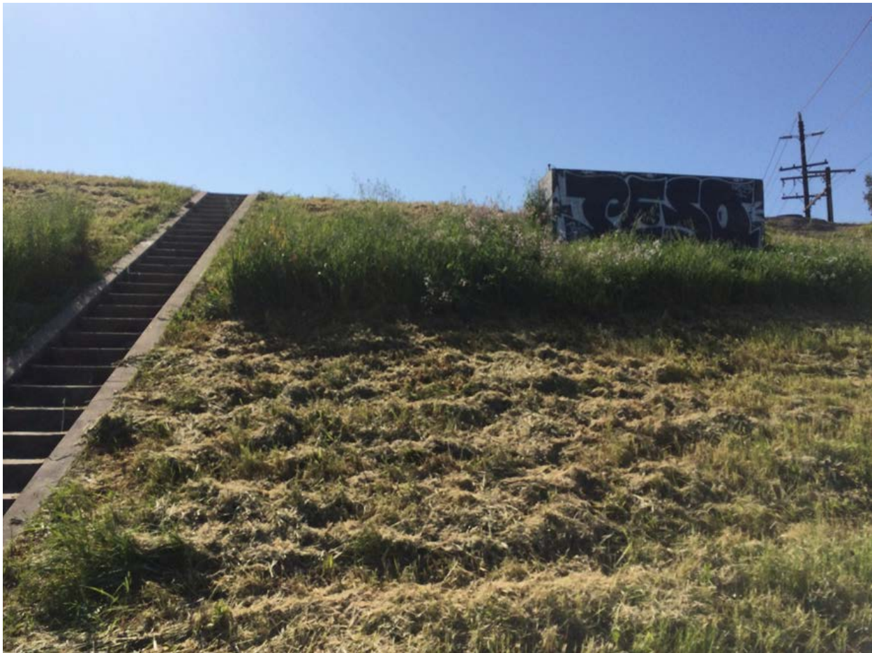
Figure 1: Waterside toe near Sump 154 looking toward levee crest
