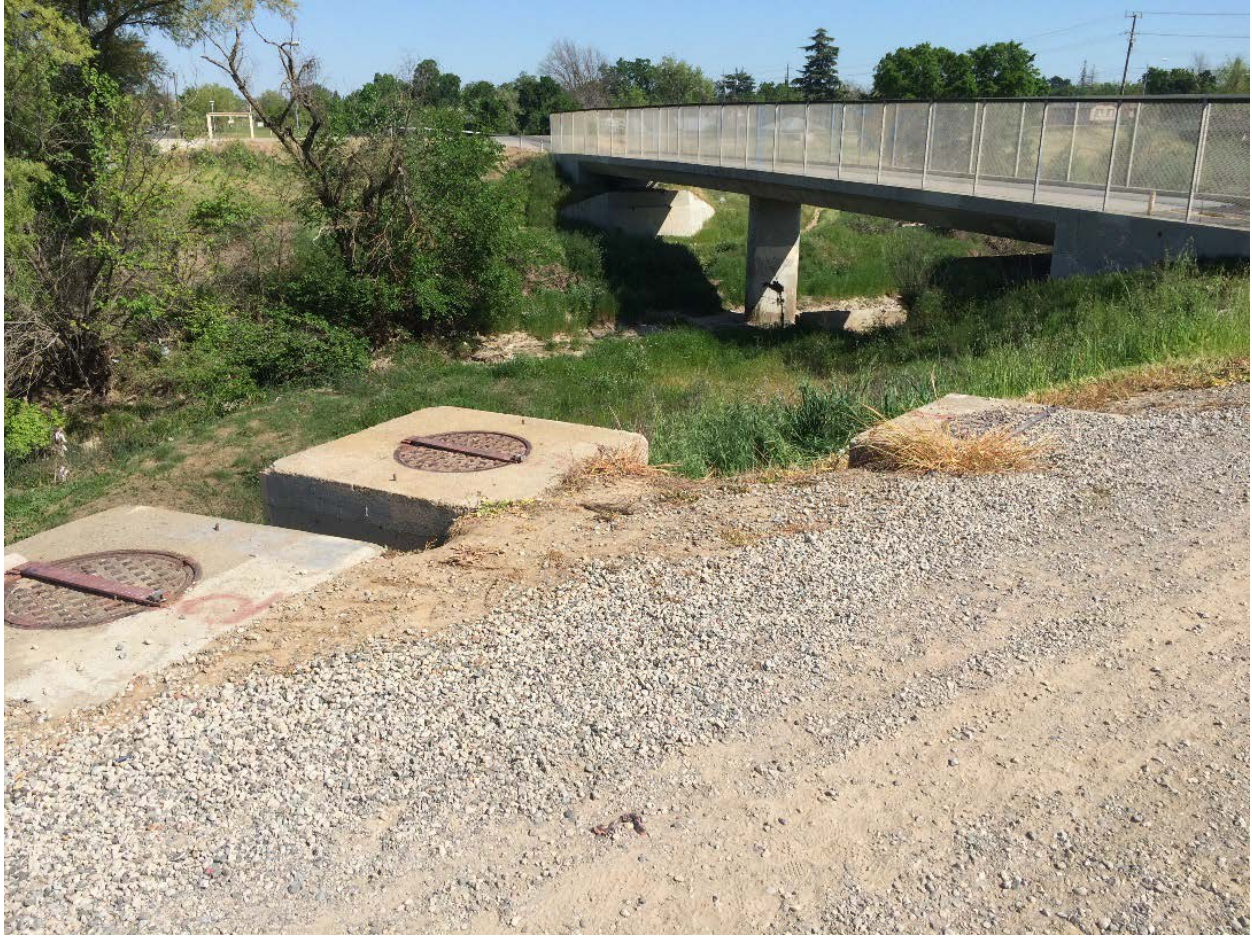
Figure 3: Siphon breaker vaults on levee crest near Sump 159
