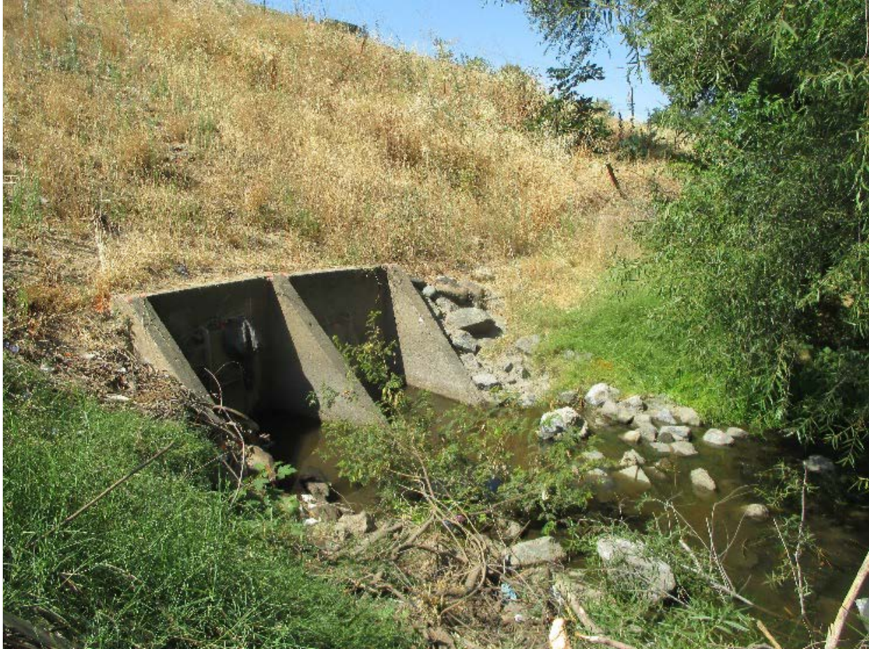
Figure 4: View looking southwest toward the Sump 159 outfall into Arcade Creek
