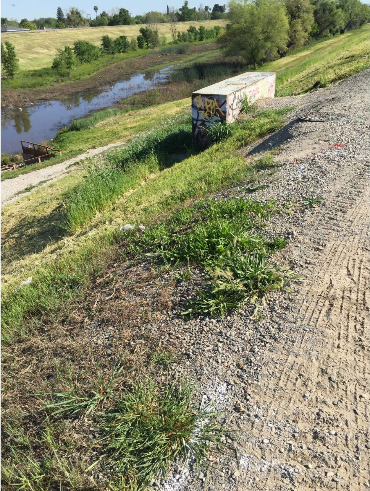
Figure 4: Waterside slope near Sump 154 looking east
