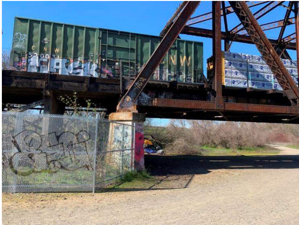
PHOTO 23: View of Pier B1, looking TT North.
