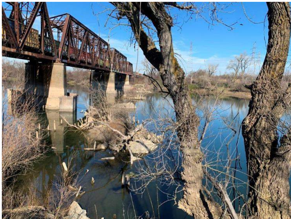
PHOTO 6: View of upstream face of bridge Segment B, looking TT East.
