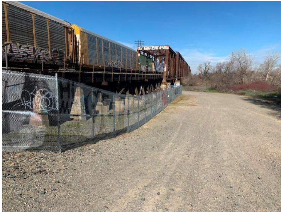
PHOTO 5: View of upstream face of bridge Segment A, looking TT East.
