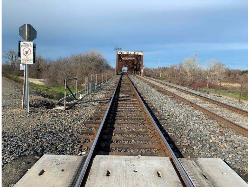
PHOTO 1: Top of Mainline 1 profile from near 92.12, looking TT East.
