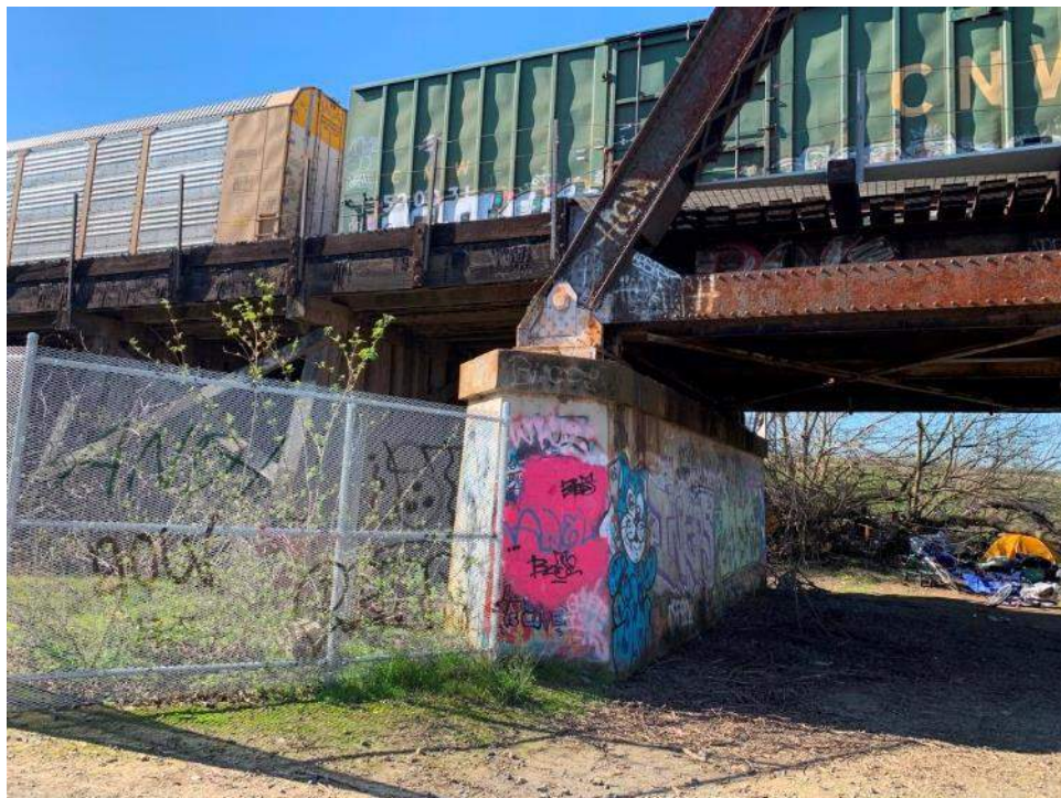
PHOTO 24: View of Pier B1, looking TT North.
