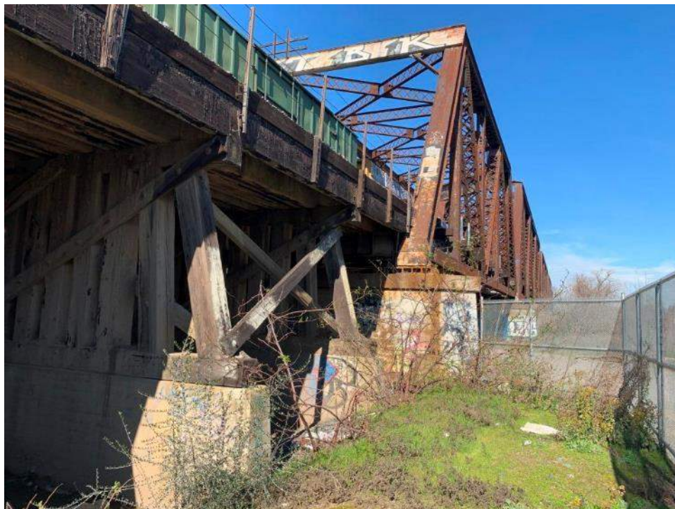
PHOTO 12: View of upstream face of Seg. A, looking TT East.
