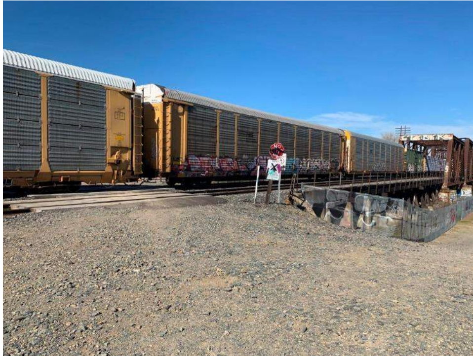
PHOTO 33: View of levee near TT West abutment, looking TT North.
