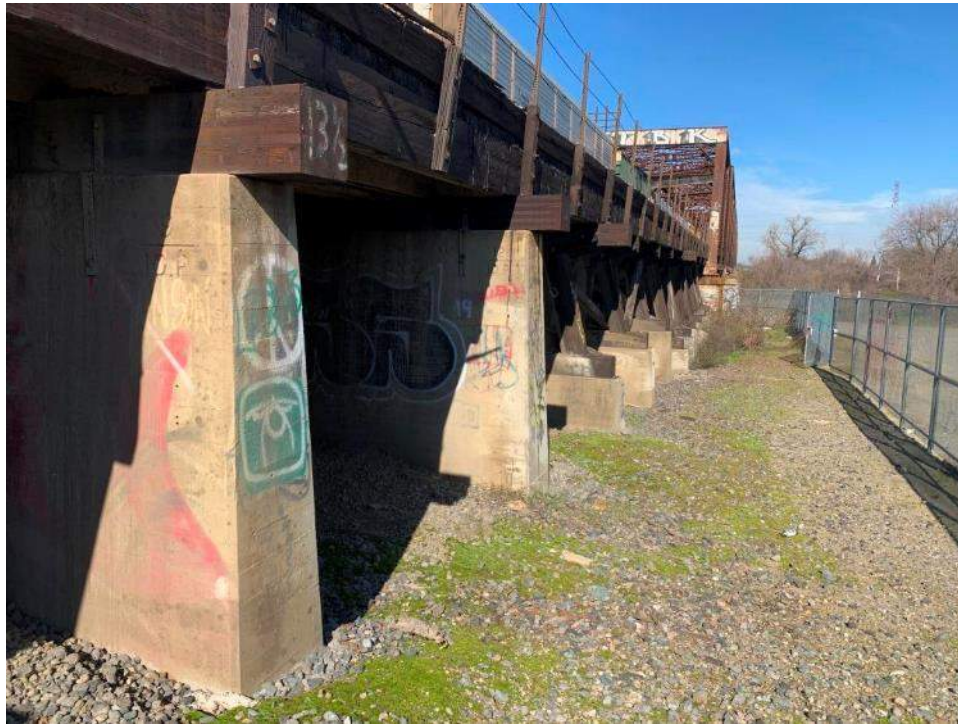
PHOTO 11: View of upstream face of Seg. A, looking TT East.
