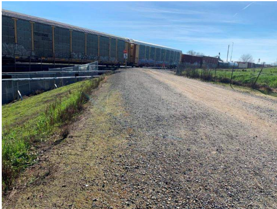
PHOTO 34: View of levee near TT West abutment, looking TT South.
