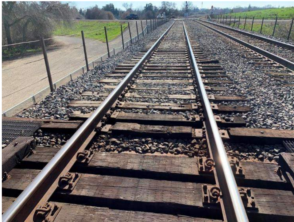
PHOTO 4: Top of Mainline 2 profile from Bridge 92.12, looking TT West.
