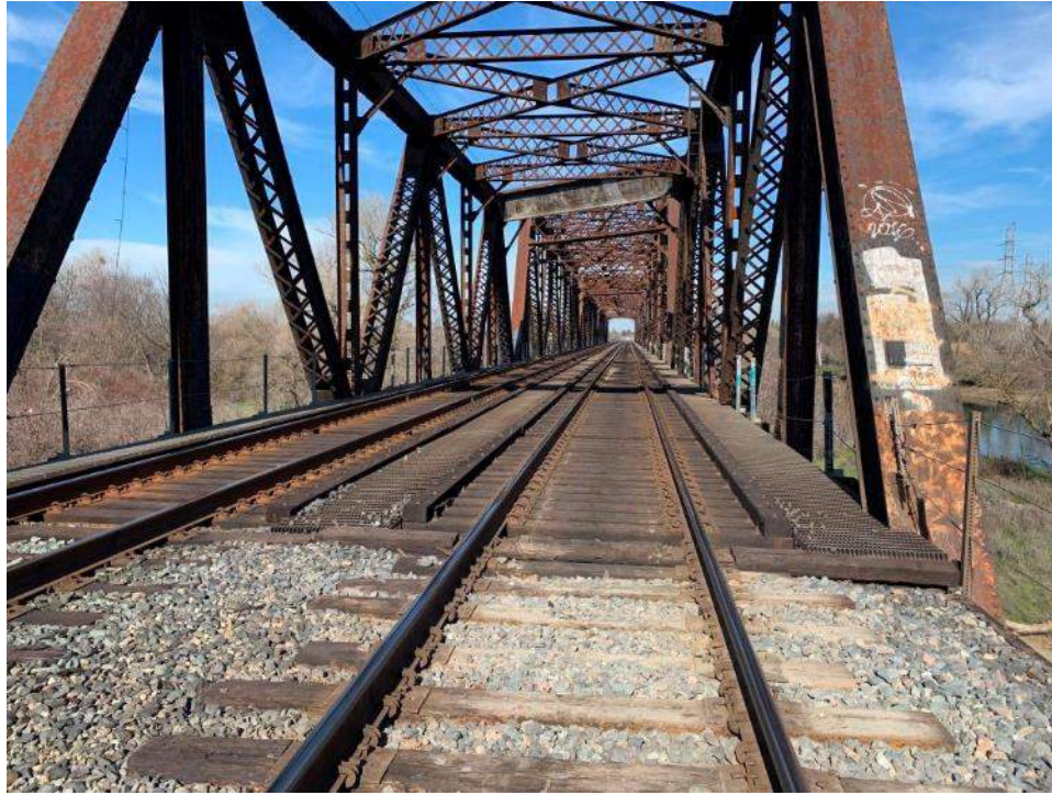
PHOTO 3: Top of Mainline 2 profile from Bridge 92.12, looking TT East.
