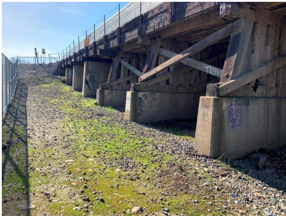
PHOTO 10: View of upstream face of Seg. A, looking TT West.
