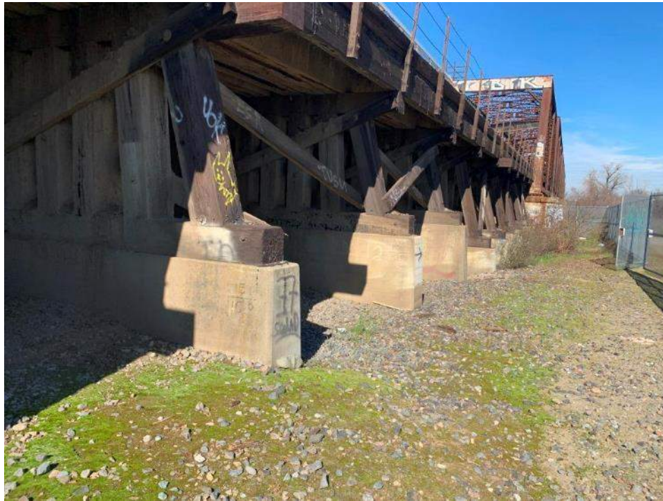
PHOTO 9: View of upstream face of Seg. A, looking TT East.
