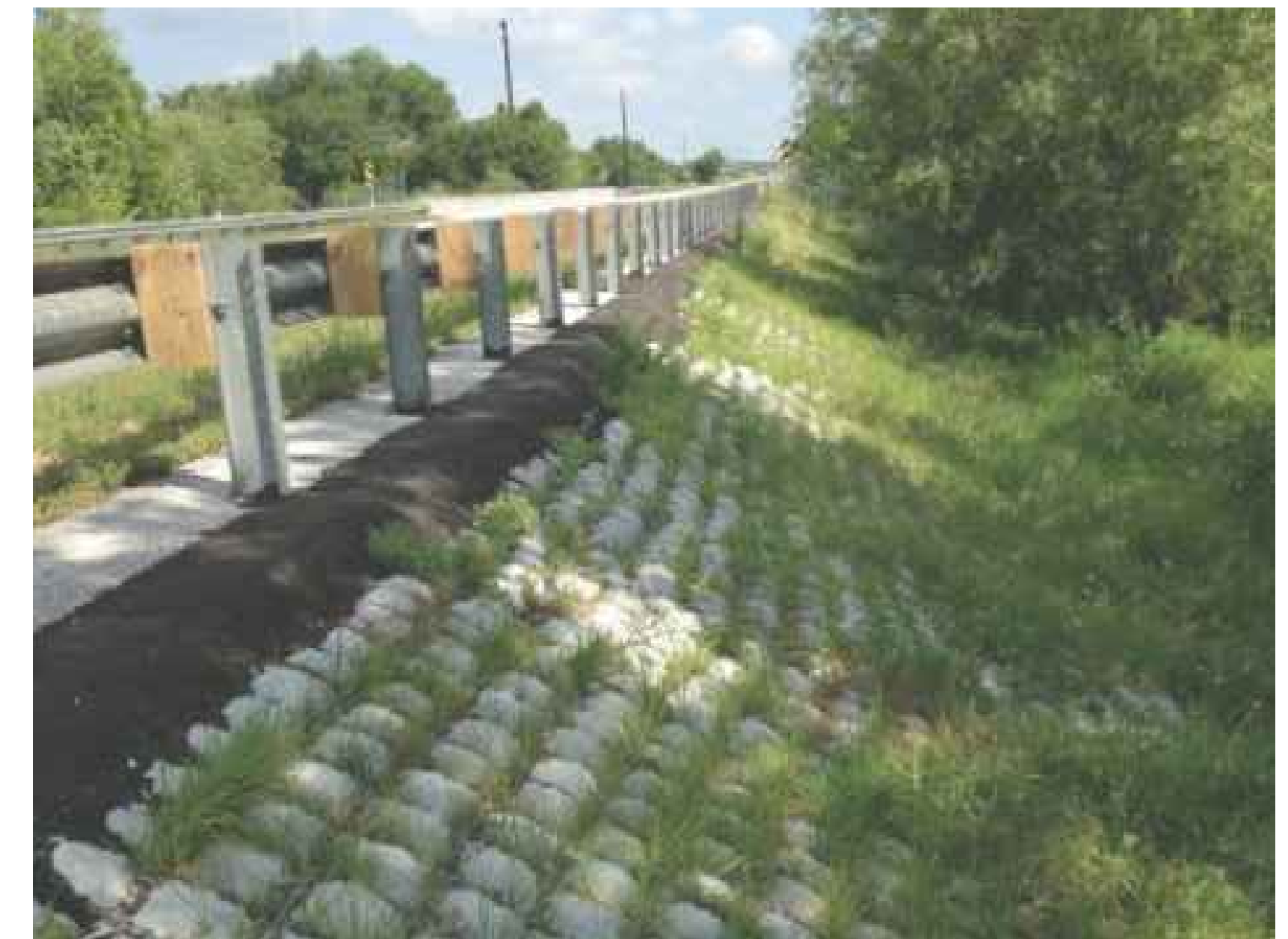
3 TYPICAL FLEXAMAT INSTALLATION
